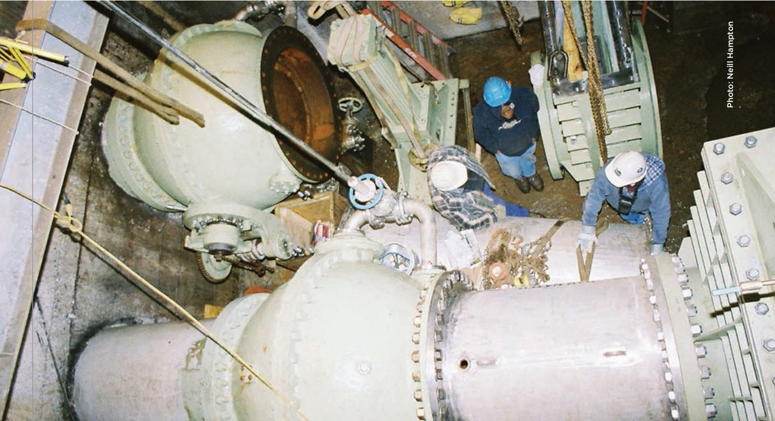
The installation of new jet flow gates.
